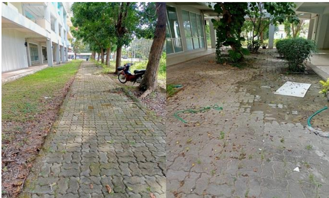
Figure 2: An example of area management using worm bricks instead of concrete pavement to allow for water permeation. The objective is to maximize the proportion of permeable area.
